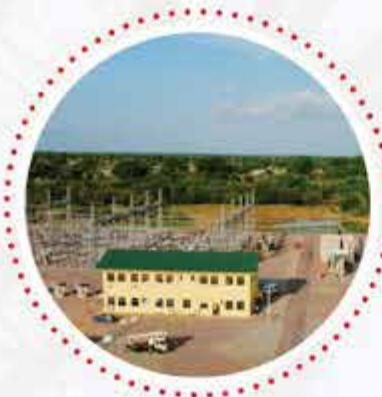
330-225kV Nayagnia Substation, Upper East Region, 2018.
